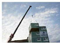
Figure 1: Prefabricated volume on ready mix concrete at the building site
